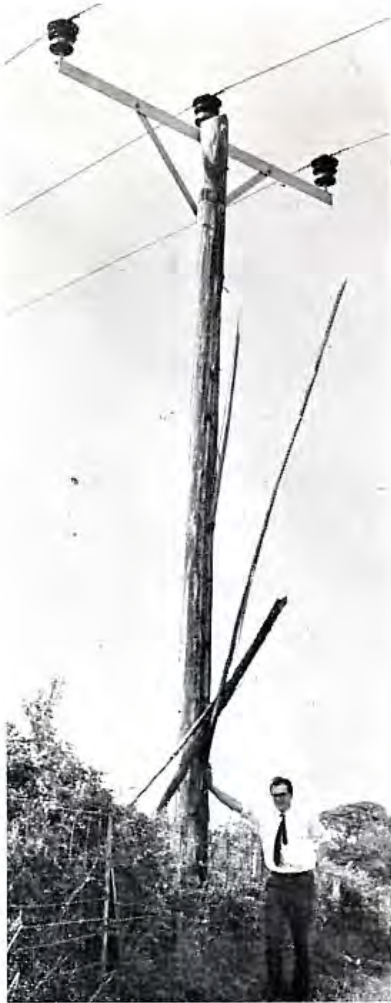
Mr. Bowen and the storm-struck pole.
