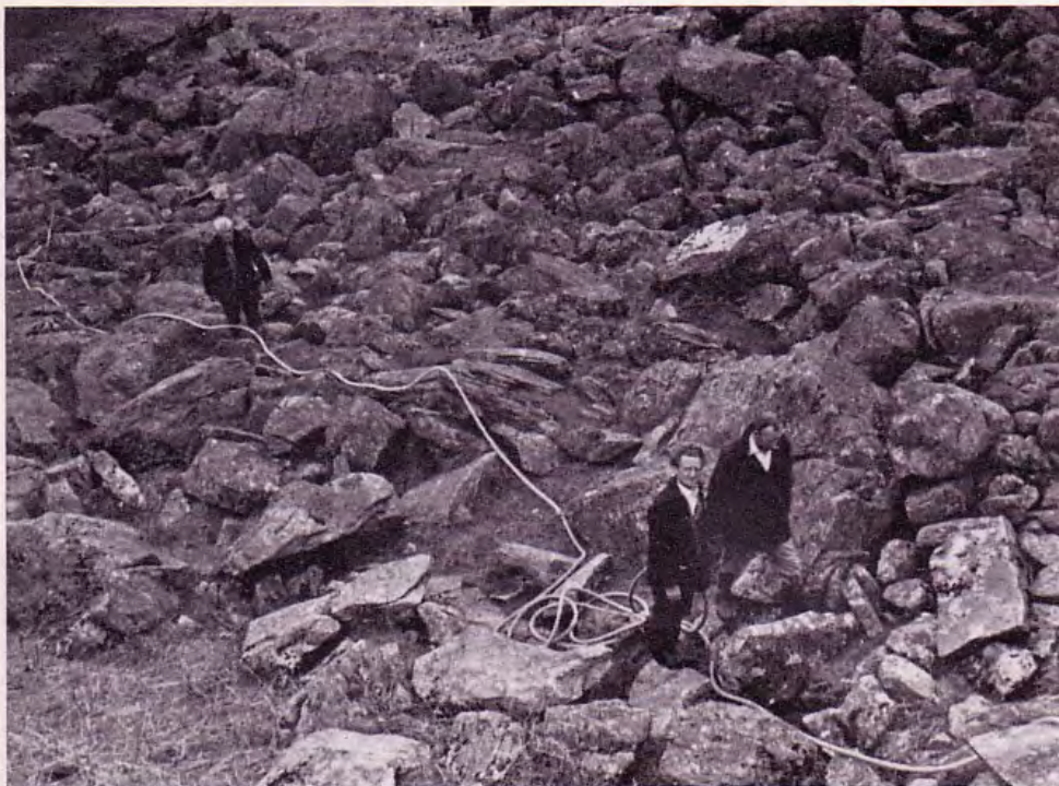
This picture shows clearly the difficult nature of the ground on which the line is being built, and explains why the raft idea was used to deliver the equipment!
